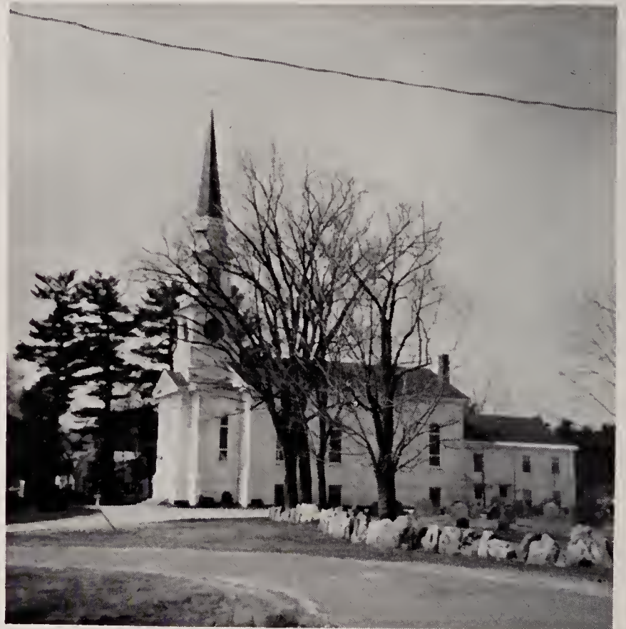
First Congregational Church erected — 1865, "Old Burying Ground" and site of first meeting house.
